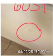
Area on wall, was filled with foam. Not properly repaired. Ruben would like to repair...
