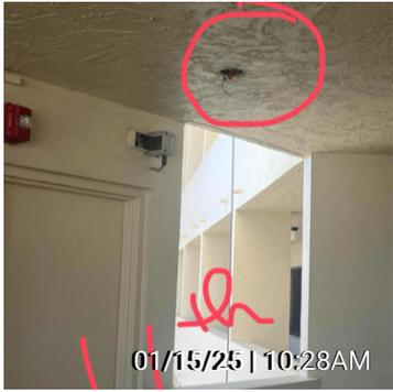
11th floor cover missing for smoke detector
