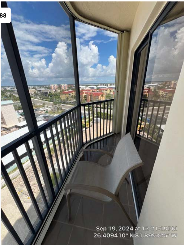
Small side balcony section of Unit 1001.
