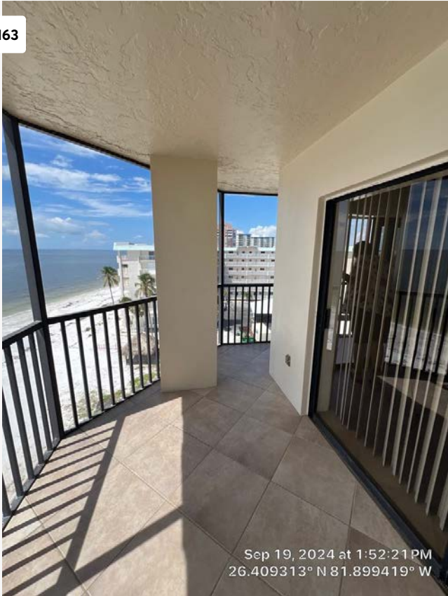
View to the north on balcony Unit 601.
