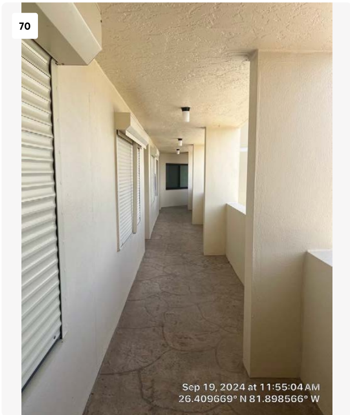
3rd floor walkway.
