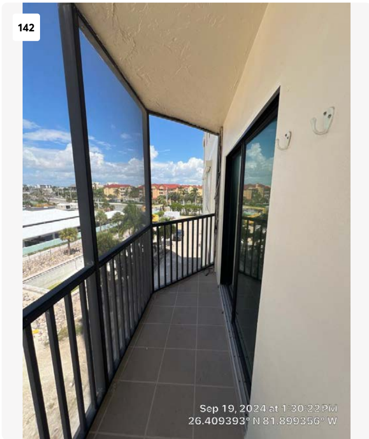
Side balcony Unit 401.
