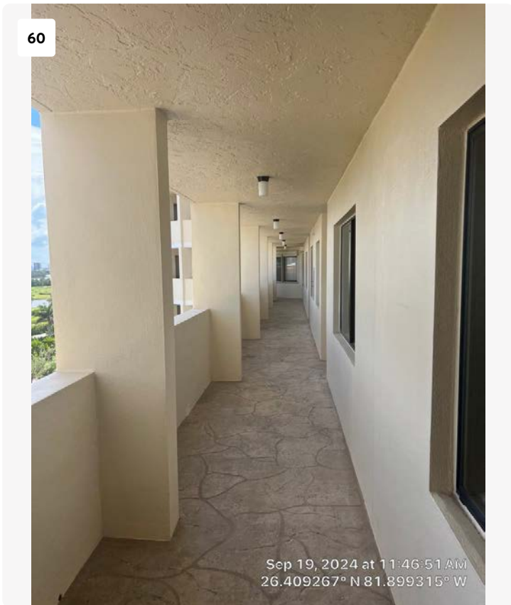
6th floor walkway.
