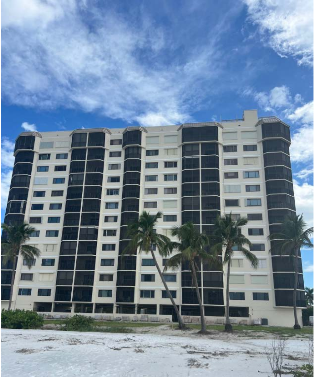
Rear Elevation - West
