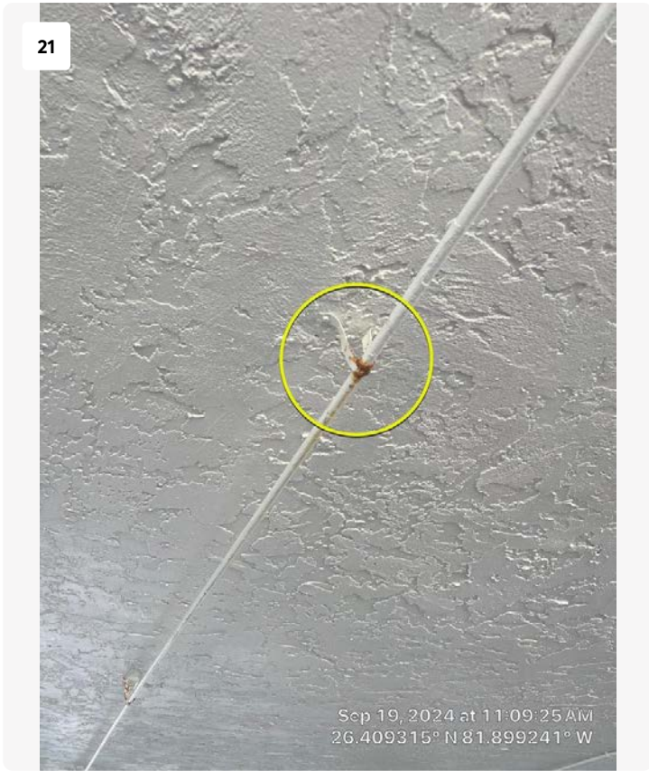
Looking east at north garage entrance. Corrosion noted on hangers. Typical of conditions throughout the garage.
