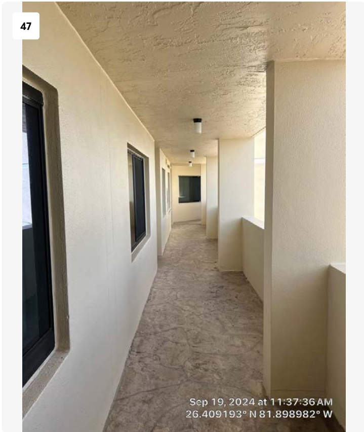
9th floor walkway.
