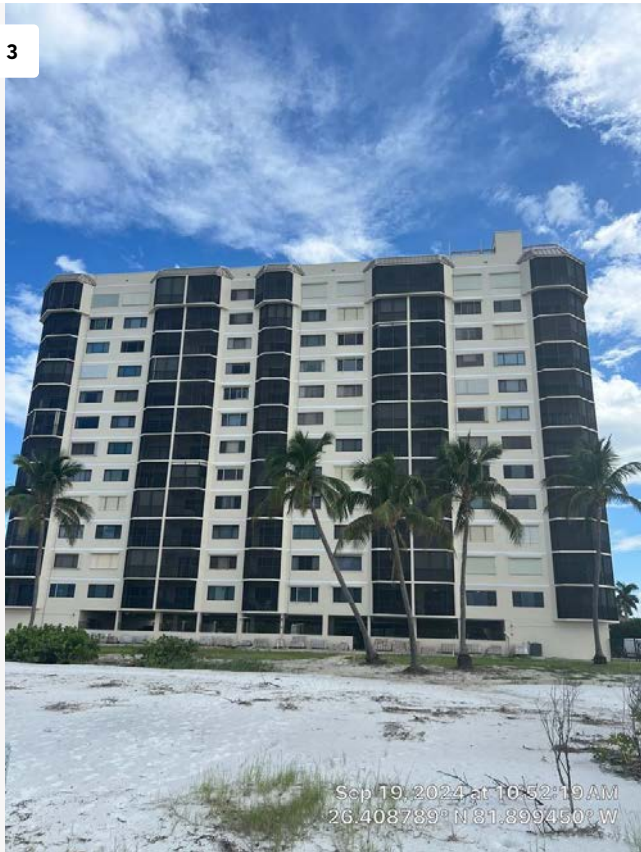
Rear elevation (west).
