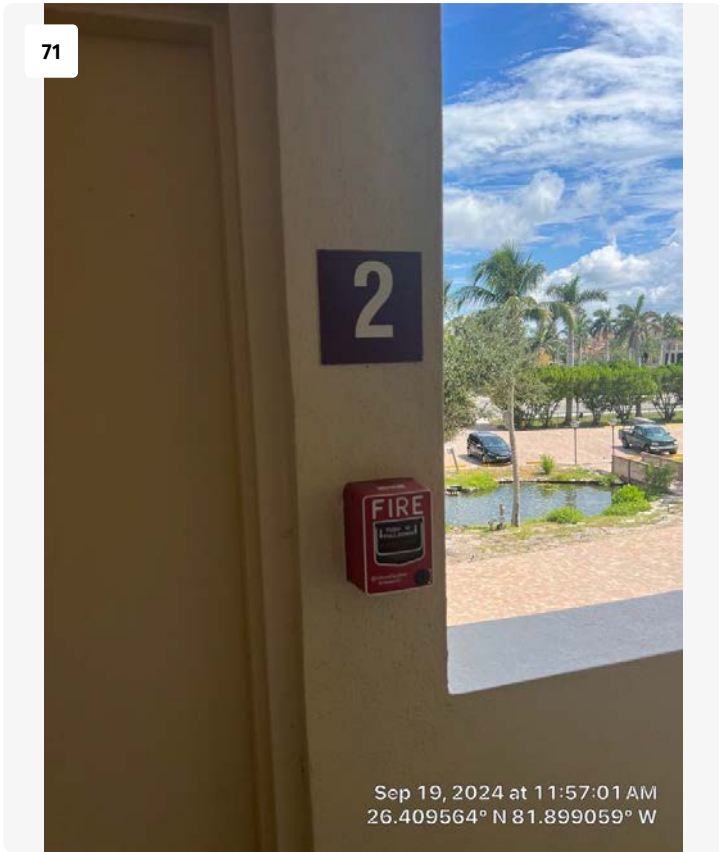
Project: Riviera Club Date: 9/19/2024, 11:57am Creator: Field Tech #1
