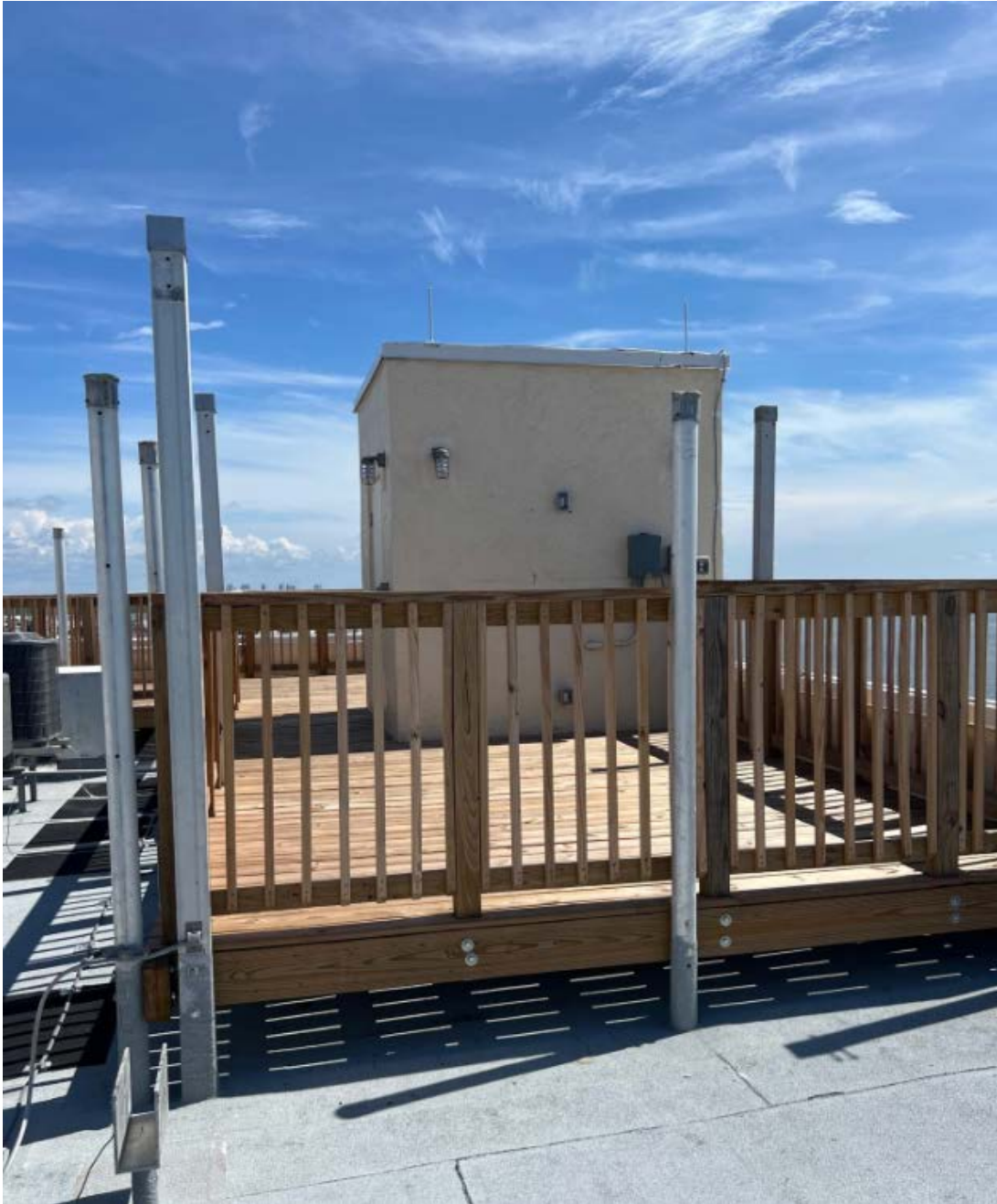
Observation Deck on Southeastern Corner-Main Roof Level
