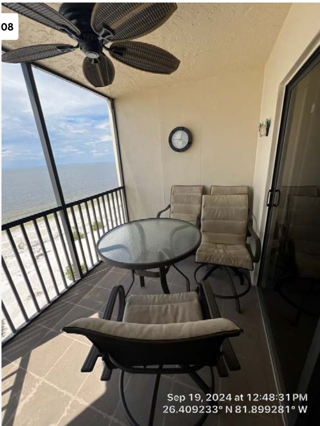
Balcony of Unit 603.
