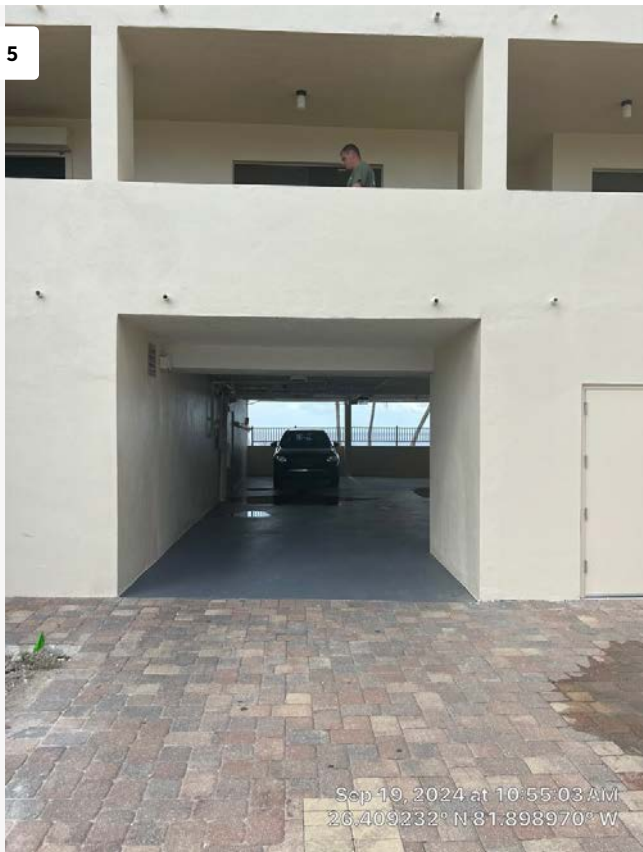
South garage entrance located on front (west) elevation.
