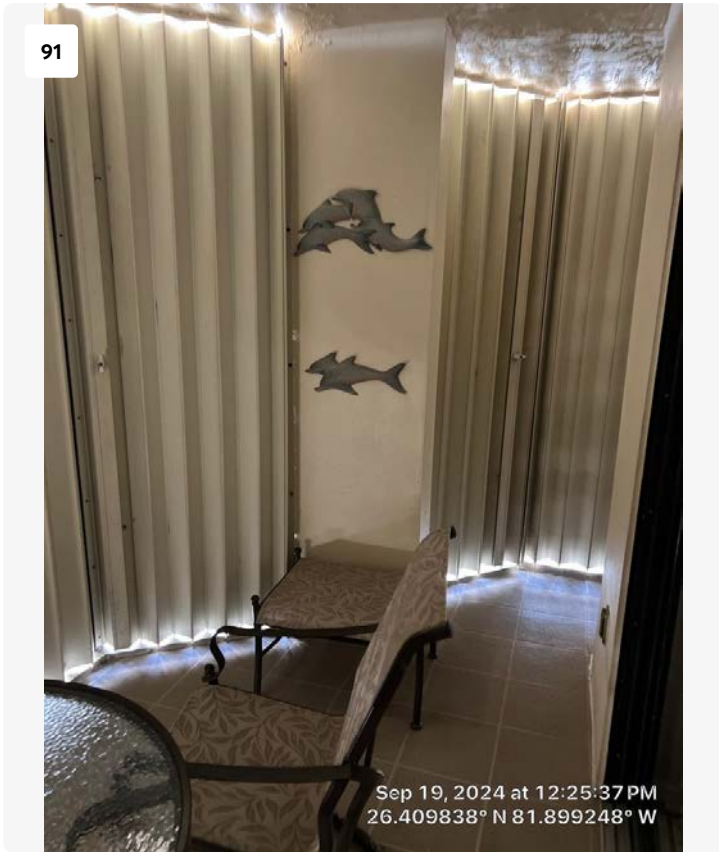
Balcony of Unit 901. Limited access to balcony slab due to tile and storm shutters.
