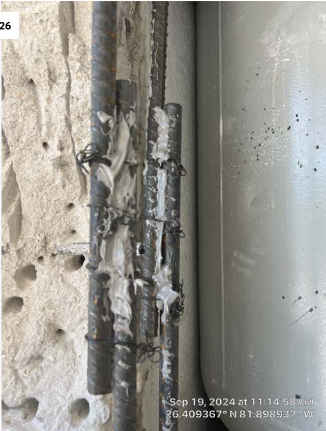
Front entrance. Concrete repair in progress
