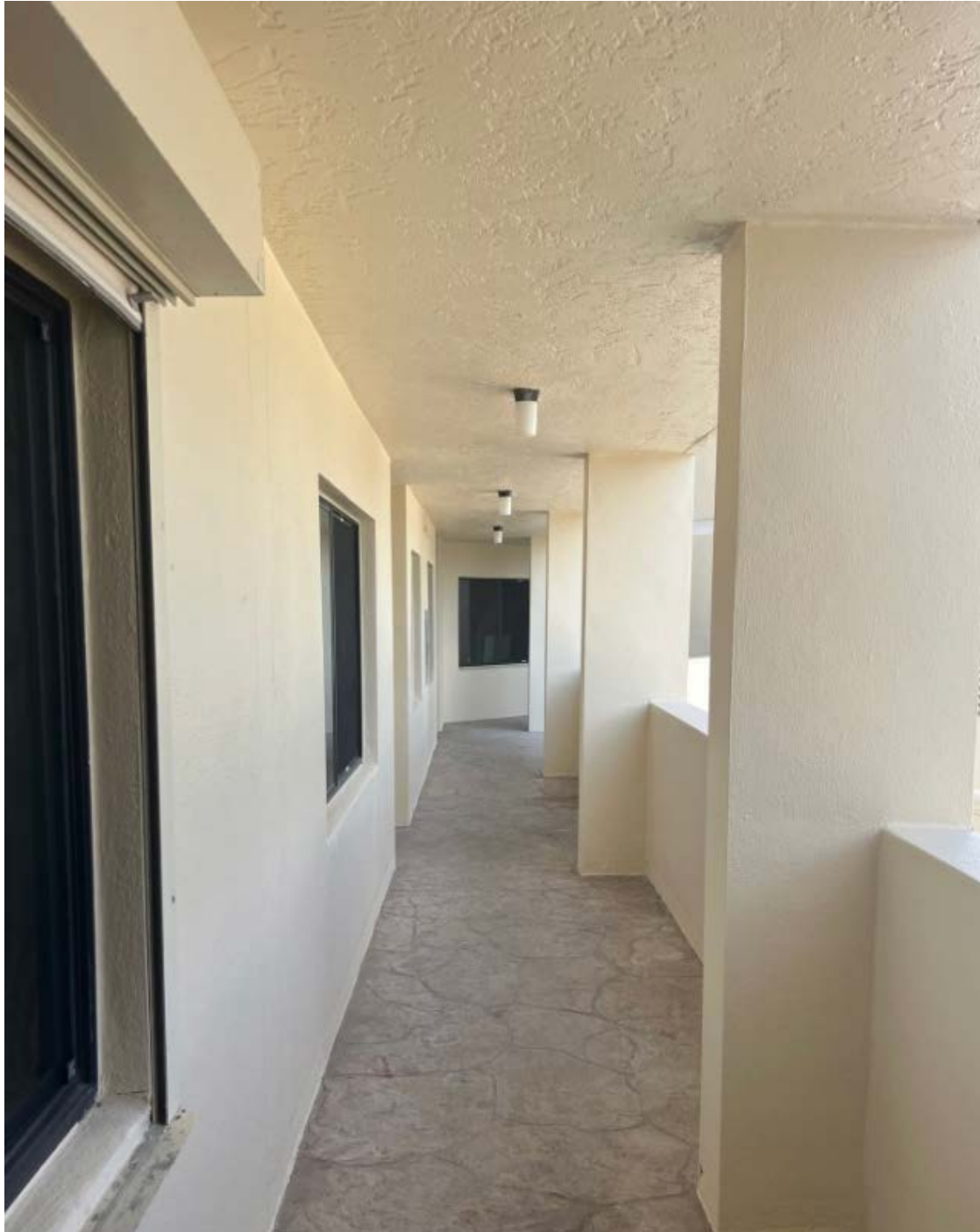
1 st Floor Walkway (typical view)
