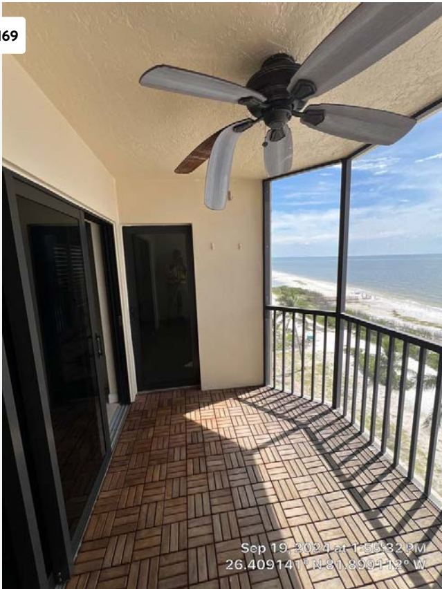
Alternate view of balcony Unit 606.
