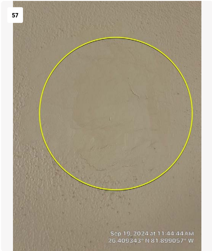
7th floor refuse chute. Previous repair noted.
