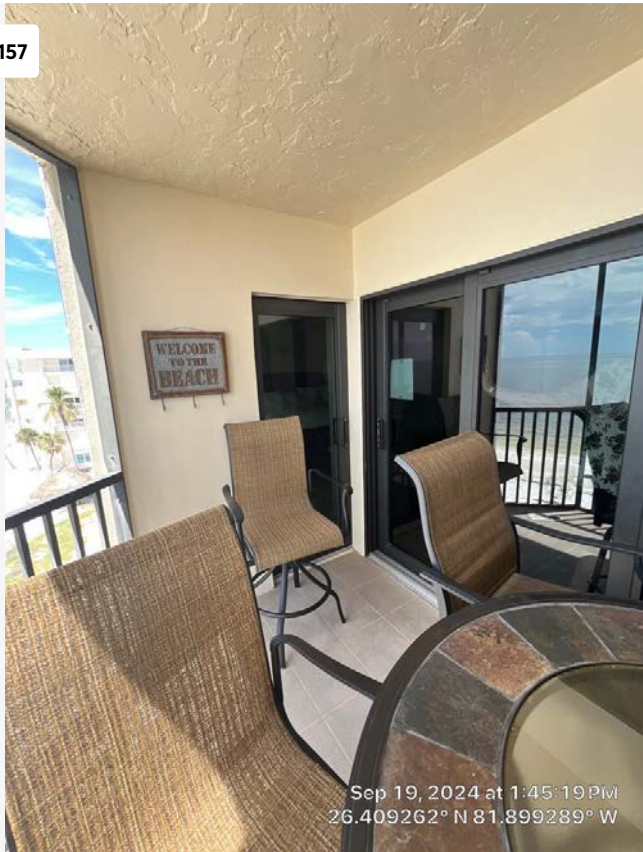
Alternate view of balcony of Unit 502.
