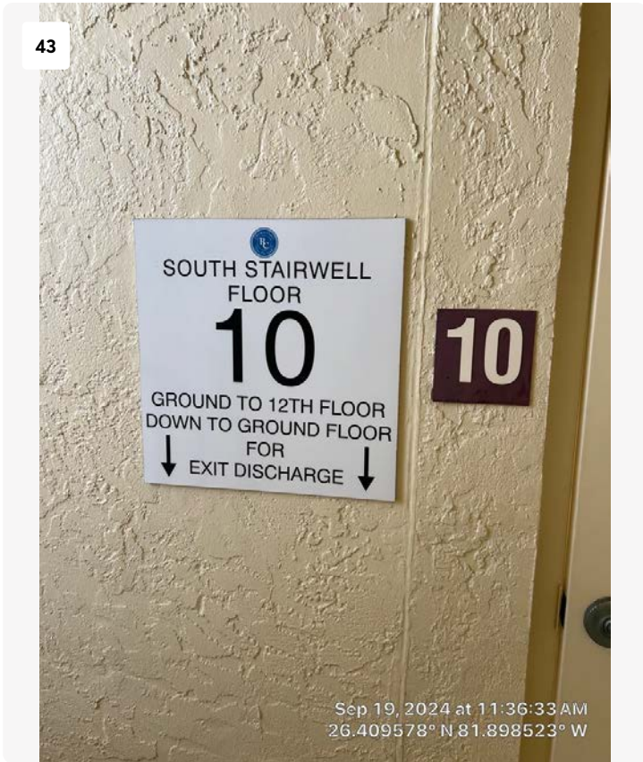
Location of damaged concrete observed on riser headed down to 9th floor.
