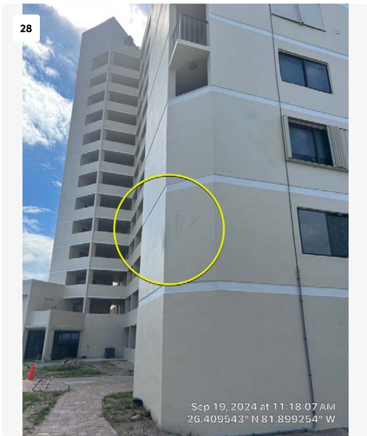
Northeastern corner of building.
