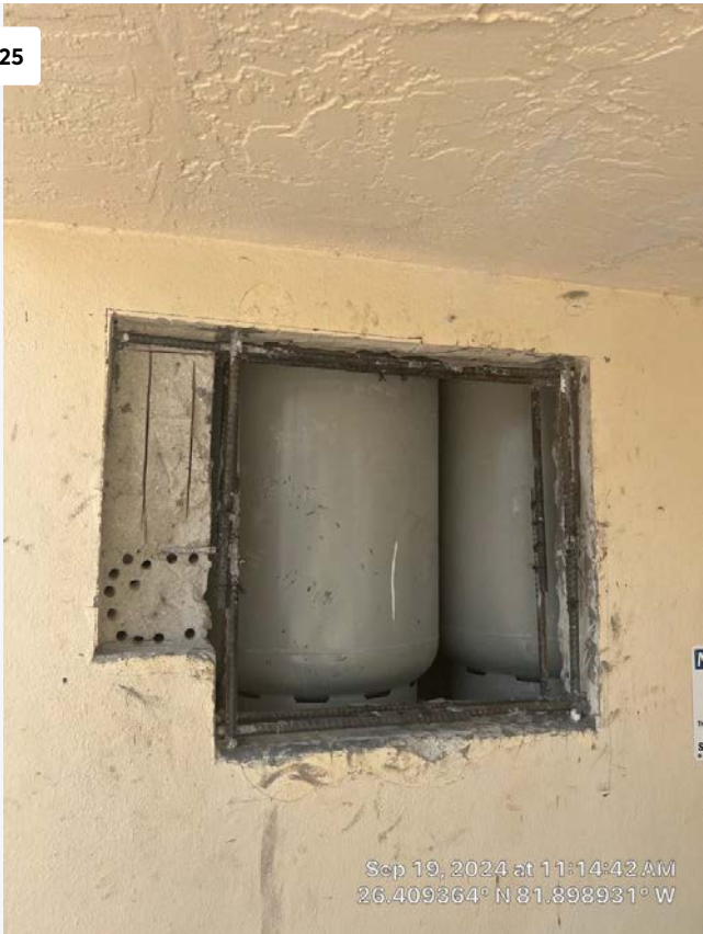
Front entrance. Concrete repair in progress
