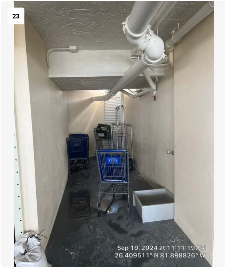
Storage area outside of interior garage elevator doors. No adverse conditions noted.
