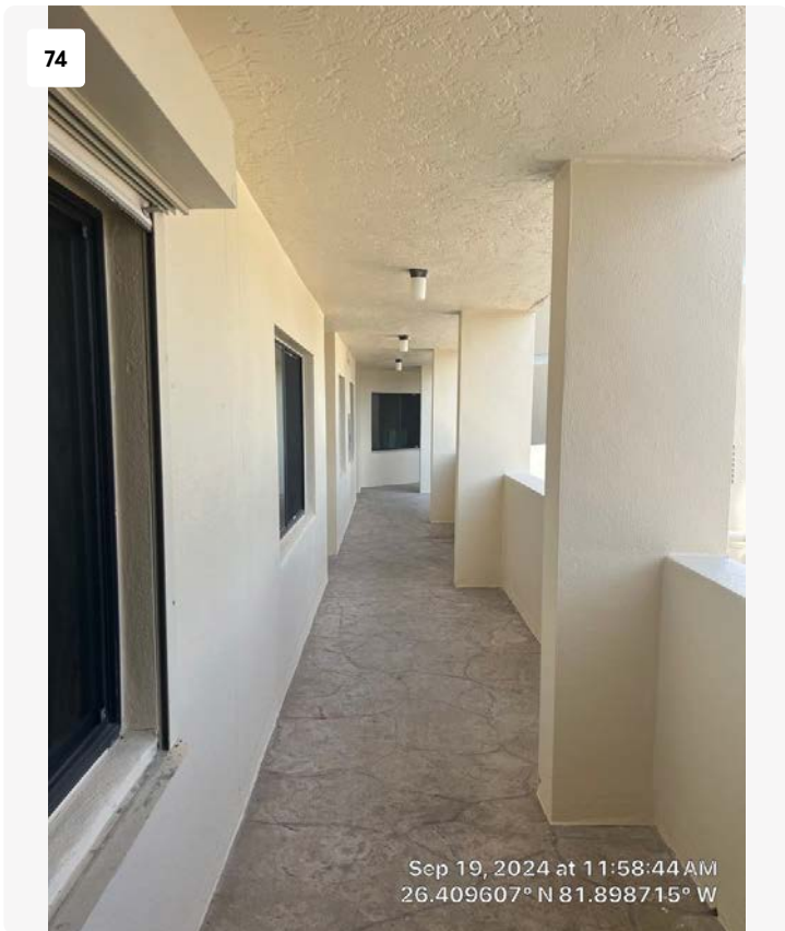
1st floor walkway.
