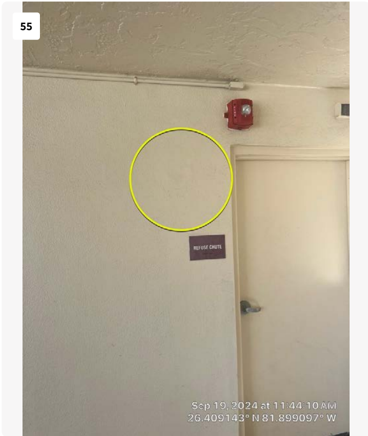
7th floor refuse chute. Previous repair noted. No action required.
