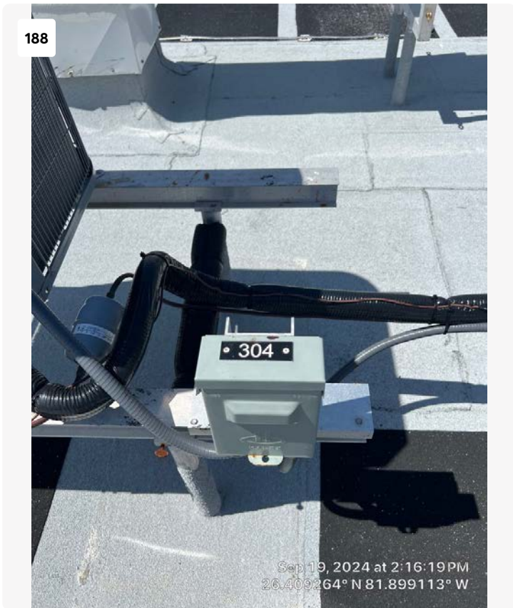
Typical of excellent conditions noted on roof of building.
