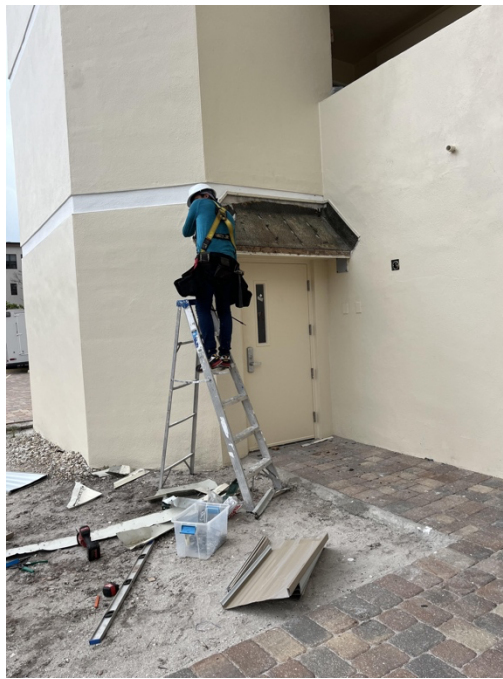
Replacing Mansard over Stair
