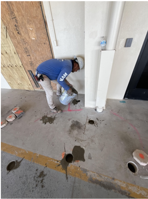
Filling voids garage floor
