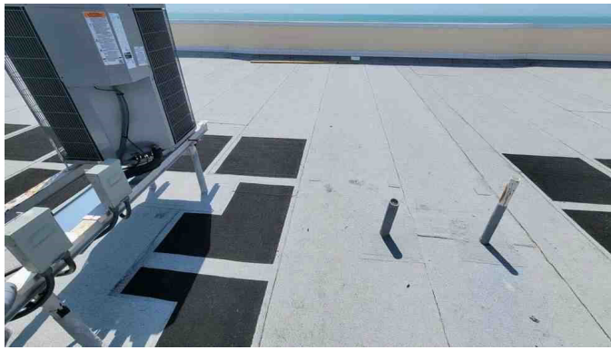
Built Up Roof
