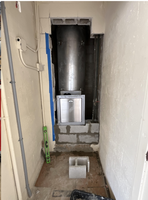
Trash room repairs
