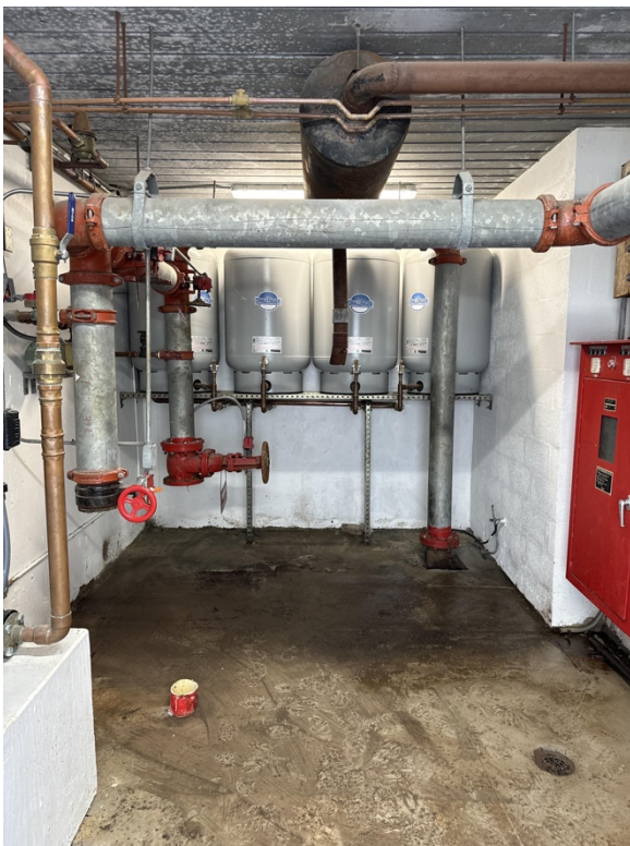
Fire Pump Room Cleared out
