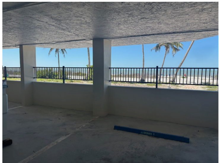
New Garage Window rails
