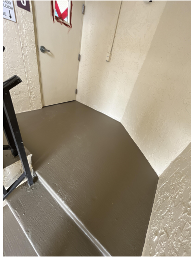
Newly painted stair landing
