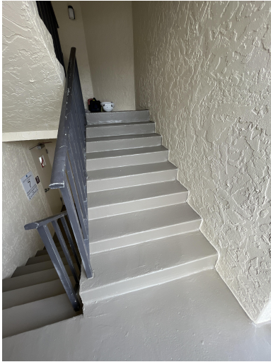
Newly painted stairs
