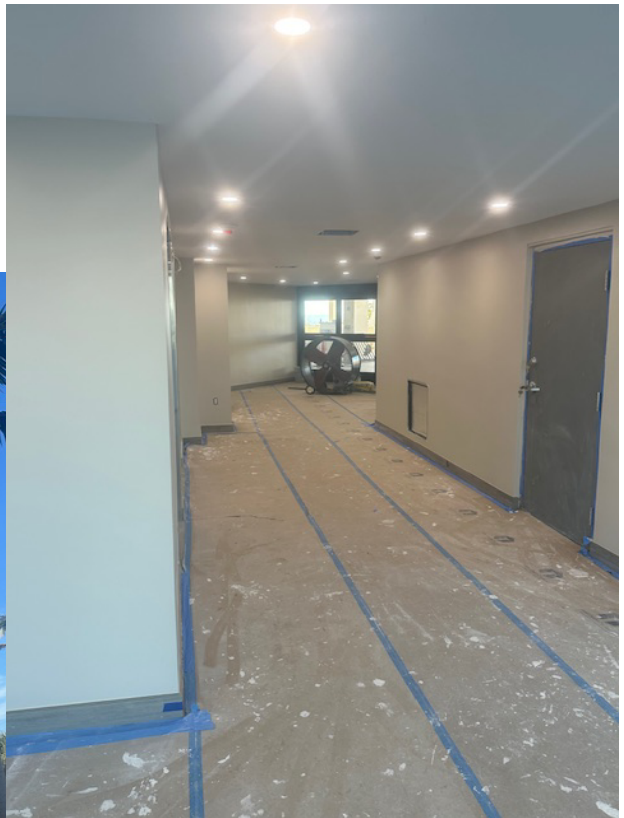
Lobby tile installed, painting underway
