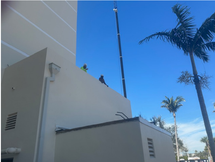
Roofers working above mech room
