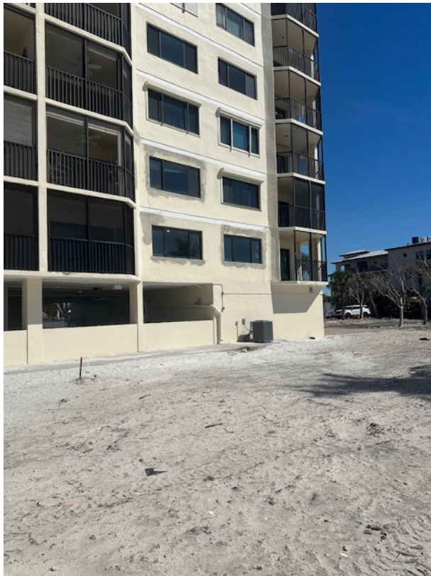
Rear paint and lanai repairs
