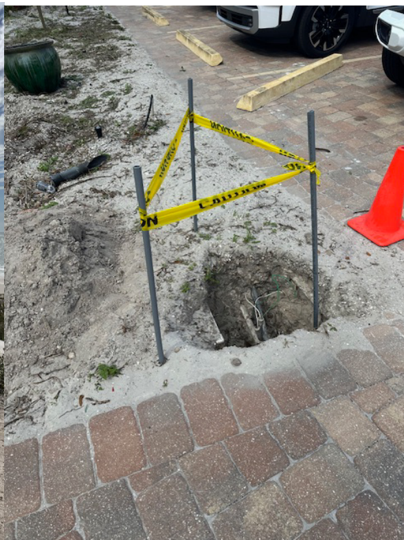
Parking lot light repairs
