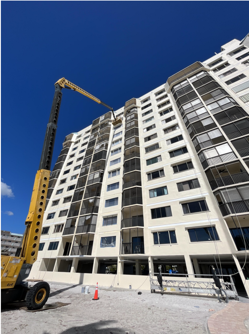
Exterior Lanai Repairs
