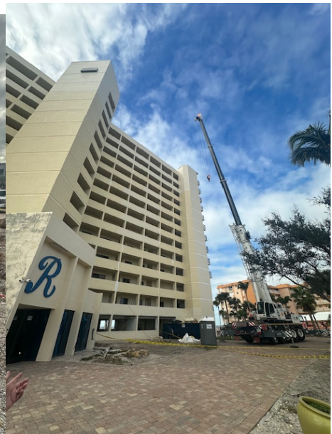
Crane Lifting Air Units
