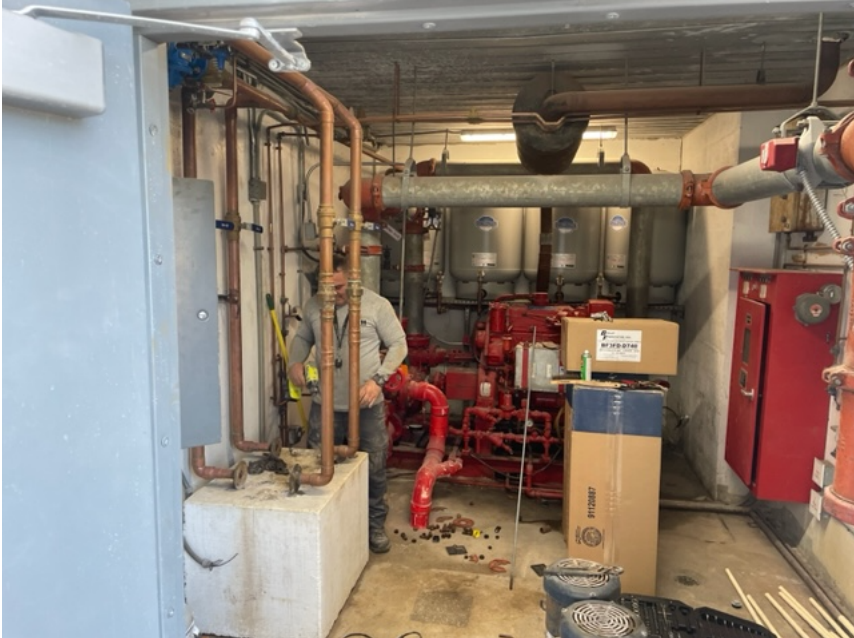
Domestic Water Pump Removal/Reinstall
