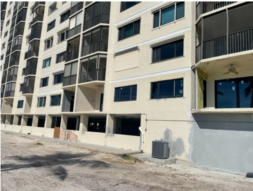
First Floor Cages Removed for Repair
