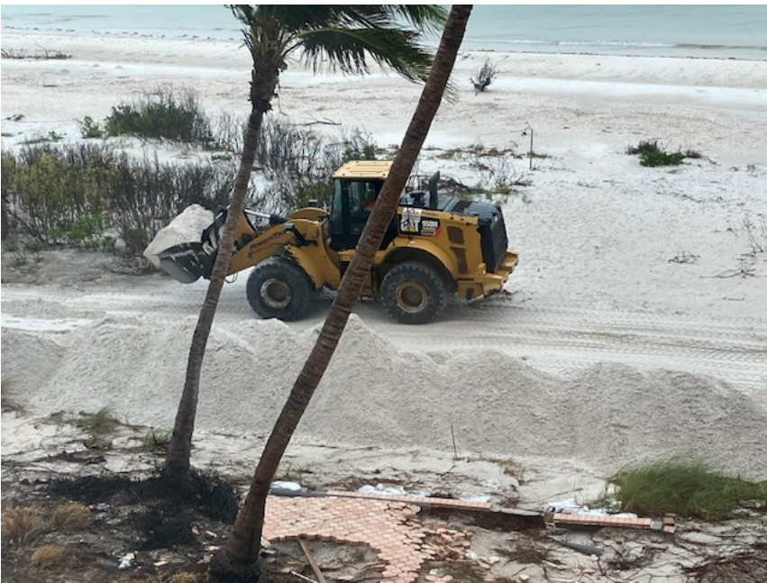
Beach Sand Bern Deposited, Not Spread Yet
