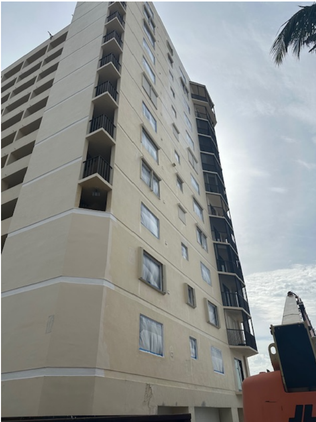
North Side Wall Being Painted
