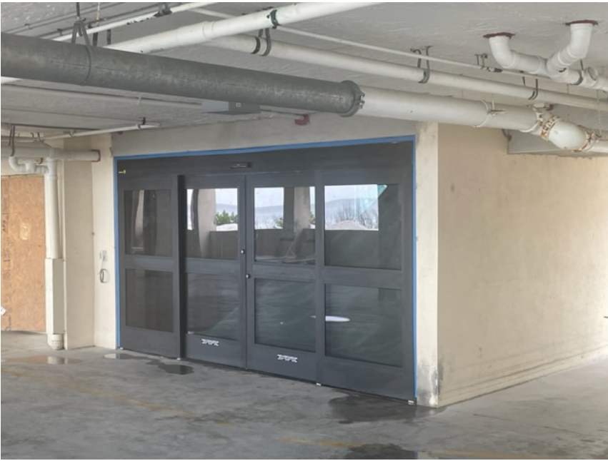
New Rear Lobby Entry Doors
