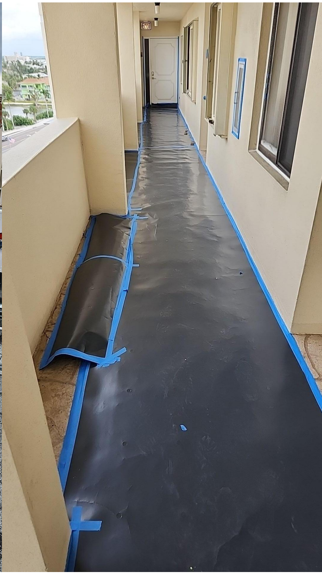
Newly Painted Front Walkway
