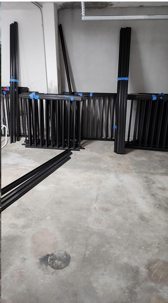
New Lanai Cage Rails for Install
