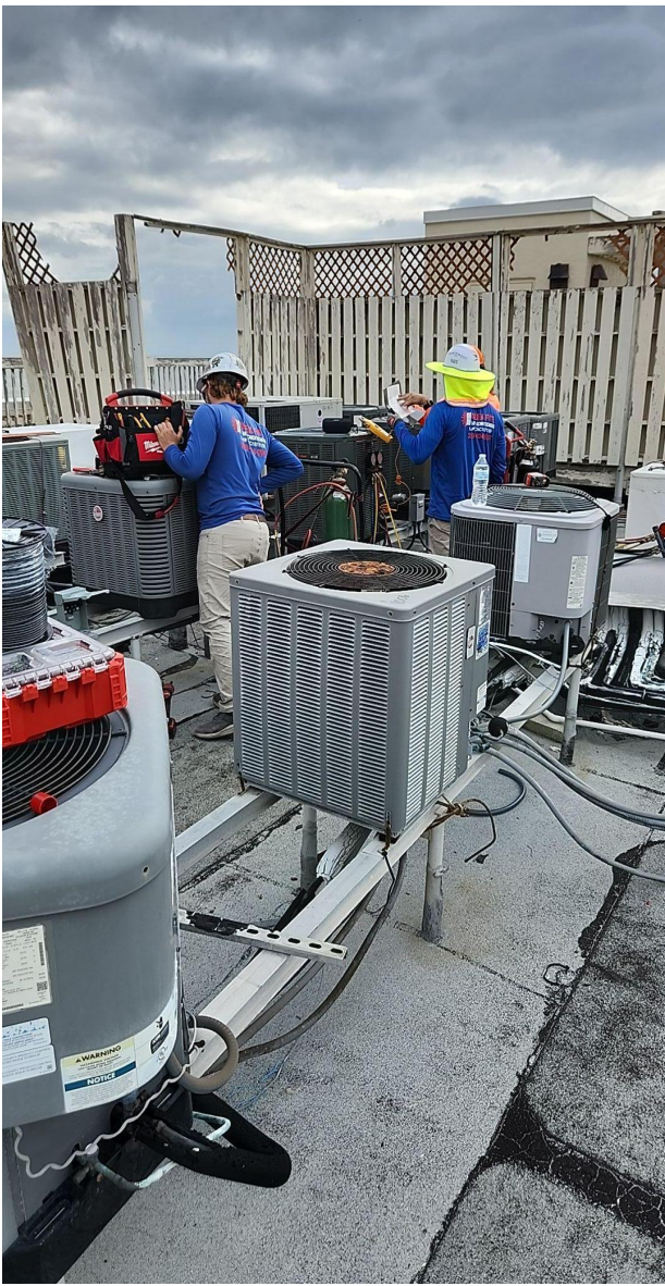
New Air Conditioner units being installed on roof
