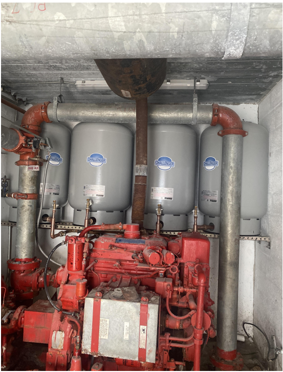
Pressure tanks installed.
