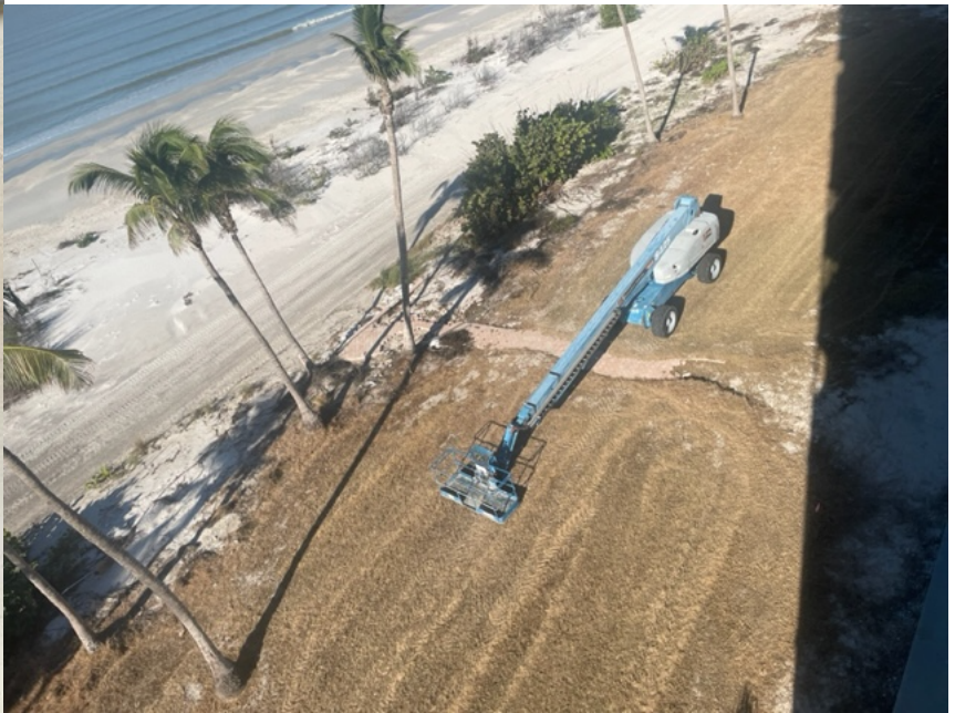
Lift to install upper floor windows.
