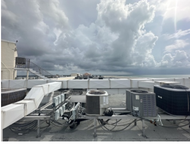
Air Conditioner Repair
