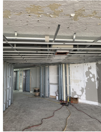
Lobby Repairs Ongoing
