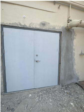
New Mechanical Room Door
