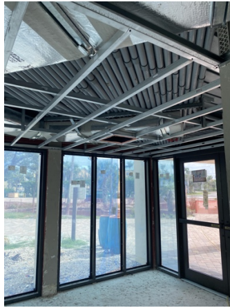
New Lobby Windows and Door
