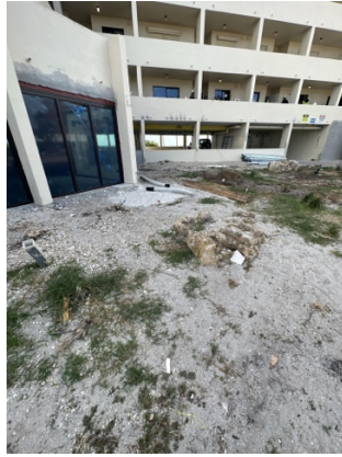
Front View Of Building
