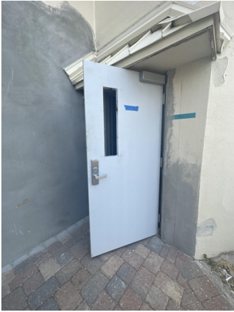
New Fire Door w/Window
