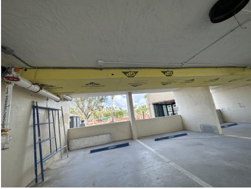
Garage Pipe Enclosure
