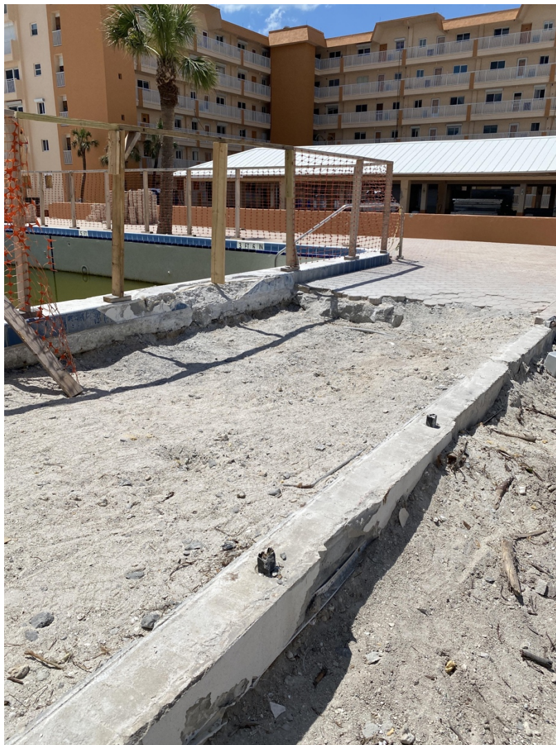
POOL ELECTRICAL PLUMBING REPAIRS
