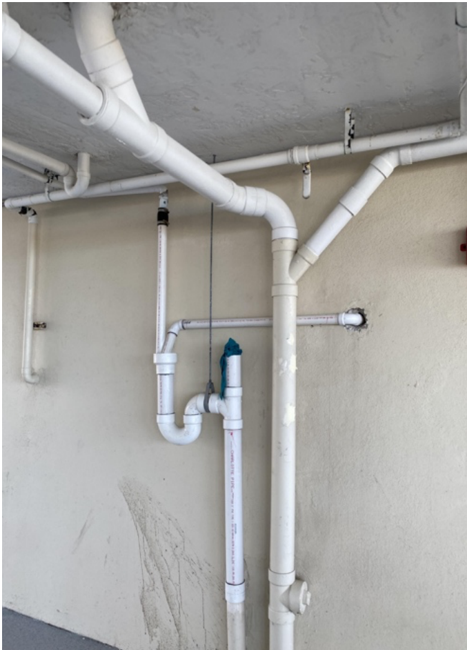
SOUTH GARAGE WALL
