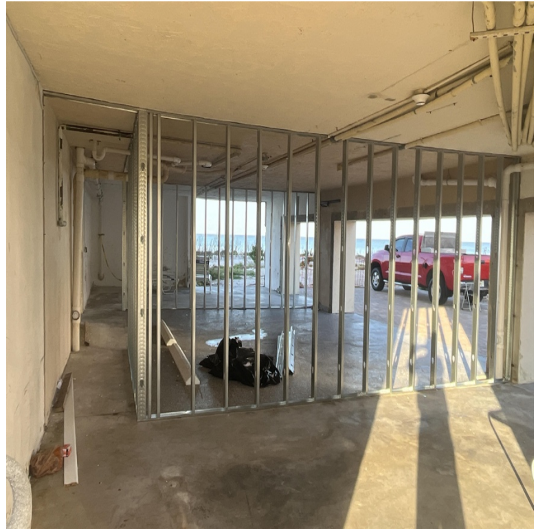
NORTH SIDE - OWNERS GARAGES.
