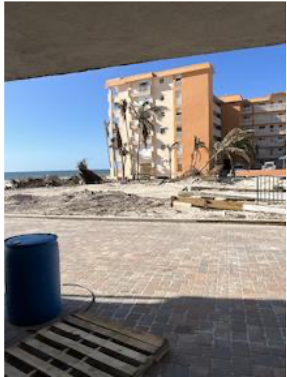
CLUBHOUSE AREA CLEARED
