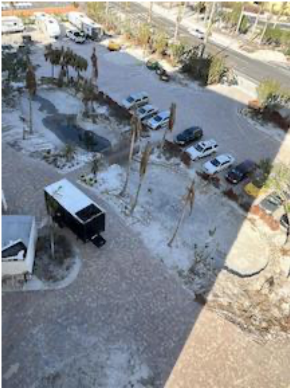
POND ROOF TOP VIEW
