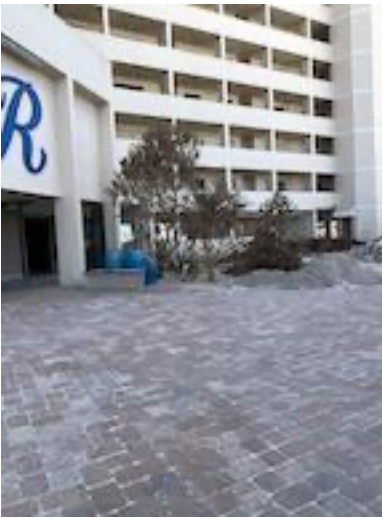
Sand Clean Up
