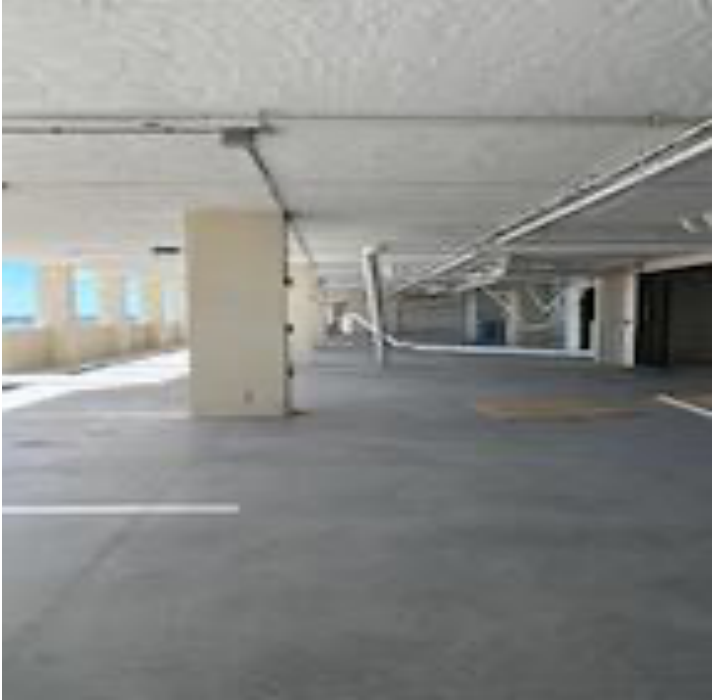
Garage After Debris Cleanup
